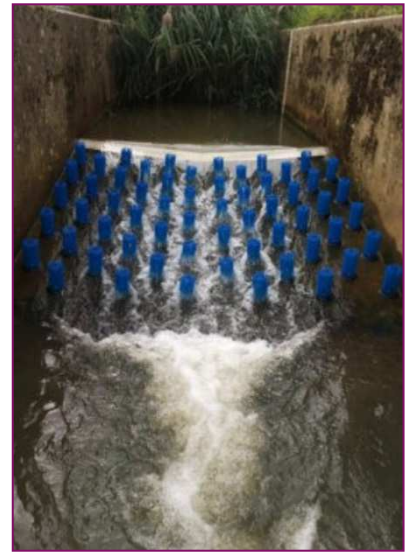
Figure 5.8 Option 7: Cylindrical Bristle Clusters on West or East Weir
